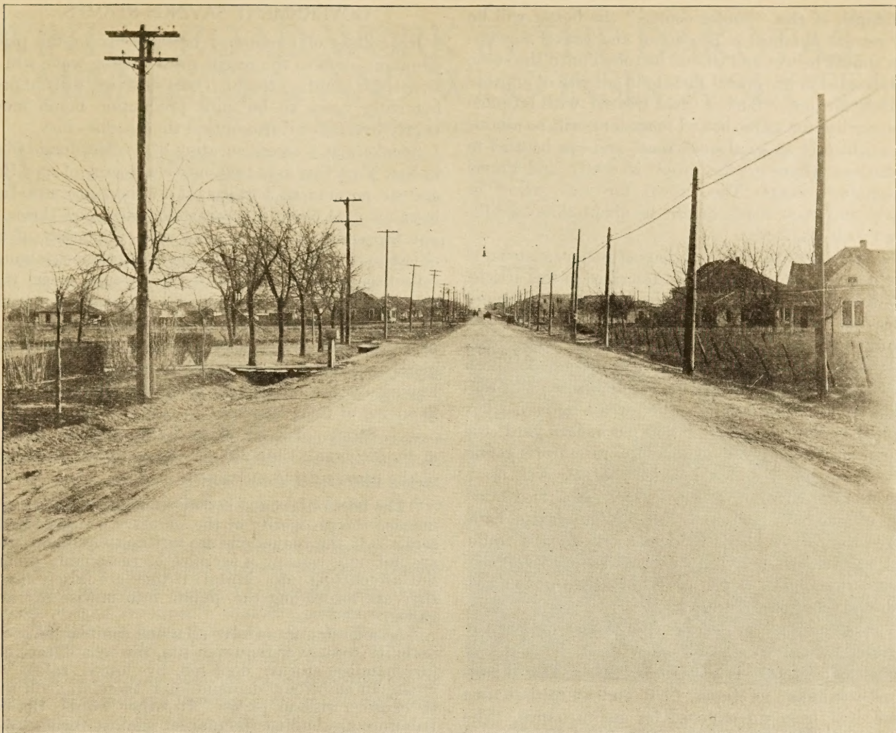
BITUMINOUS TREATED WATER-BOUND MACADAM ROAD IN TEXAS. PHOTOGRAPH TAKEN THREE YEARS AFTER CONSTRUCTION.
